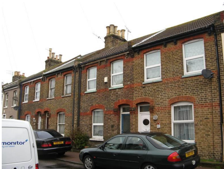
No. 19 Brockley Road (on left) is one of the few houses to retain its original windows
