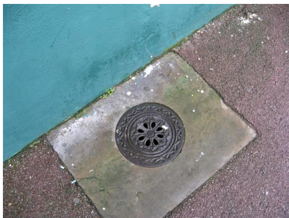
Cast iron coal hole in Grotto Road
